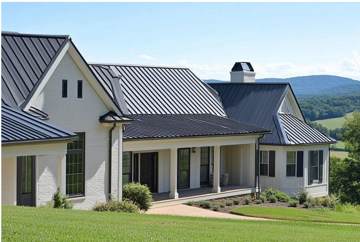
A metal roof is a one-time investment that outlasts the typical asphalt roof by 3 to 4 cycles.
