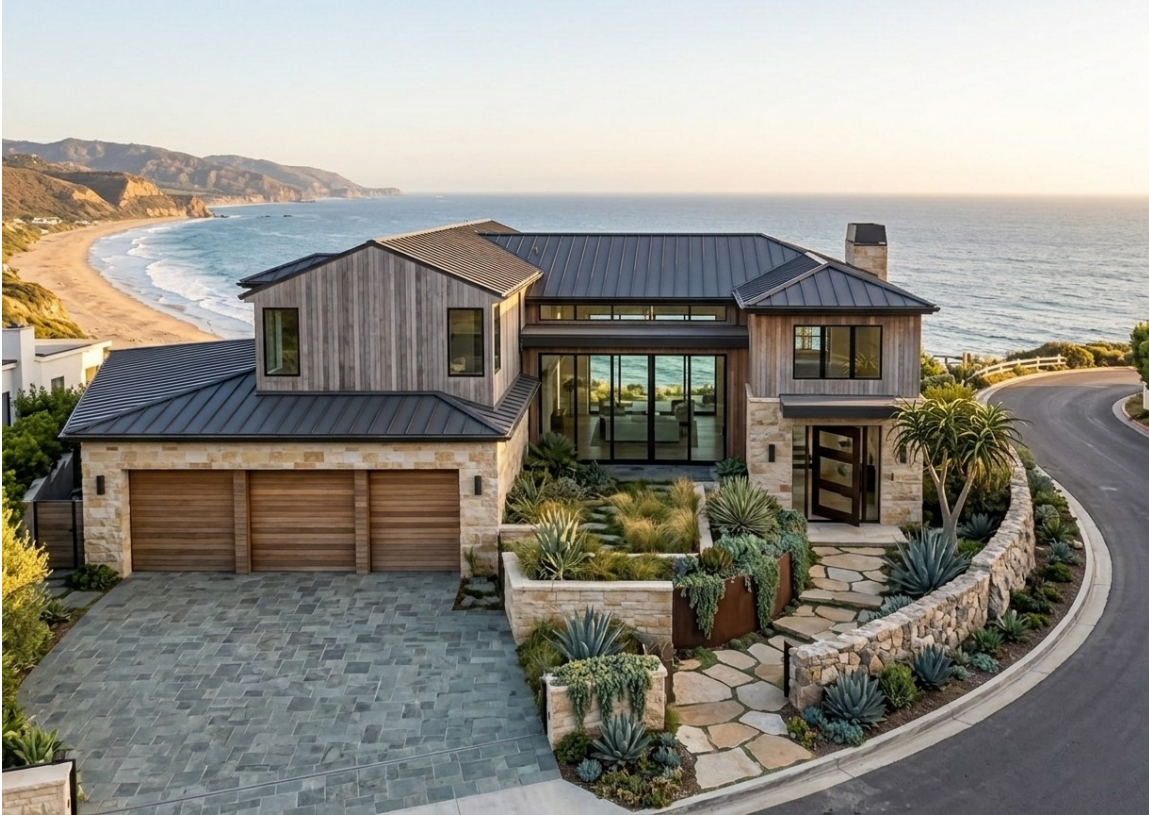
Standing seam installation in Malibu, aluminum panels, PVDF coating, full marine-grade flashing.
