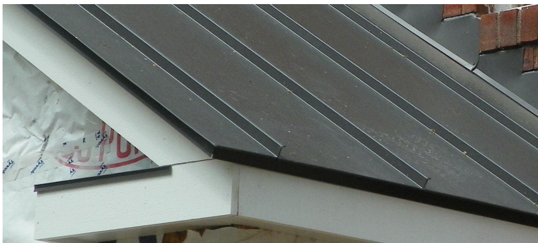
Detail shot of mechanically formed standing seam, note the crisp, continuous fold.
