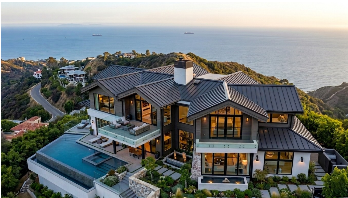
Aluminum standing seam on a Malibu home, built for salt air, sun, and ocean wind.
