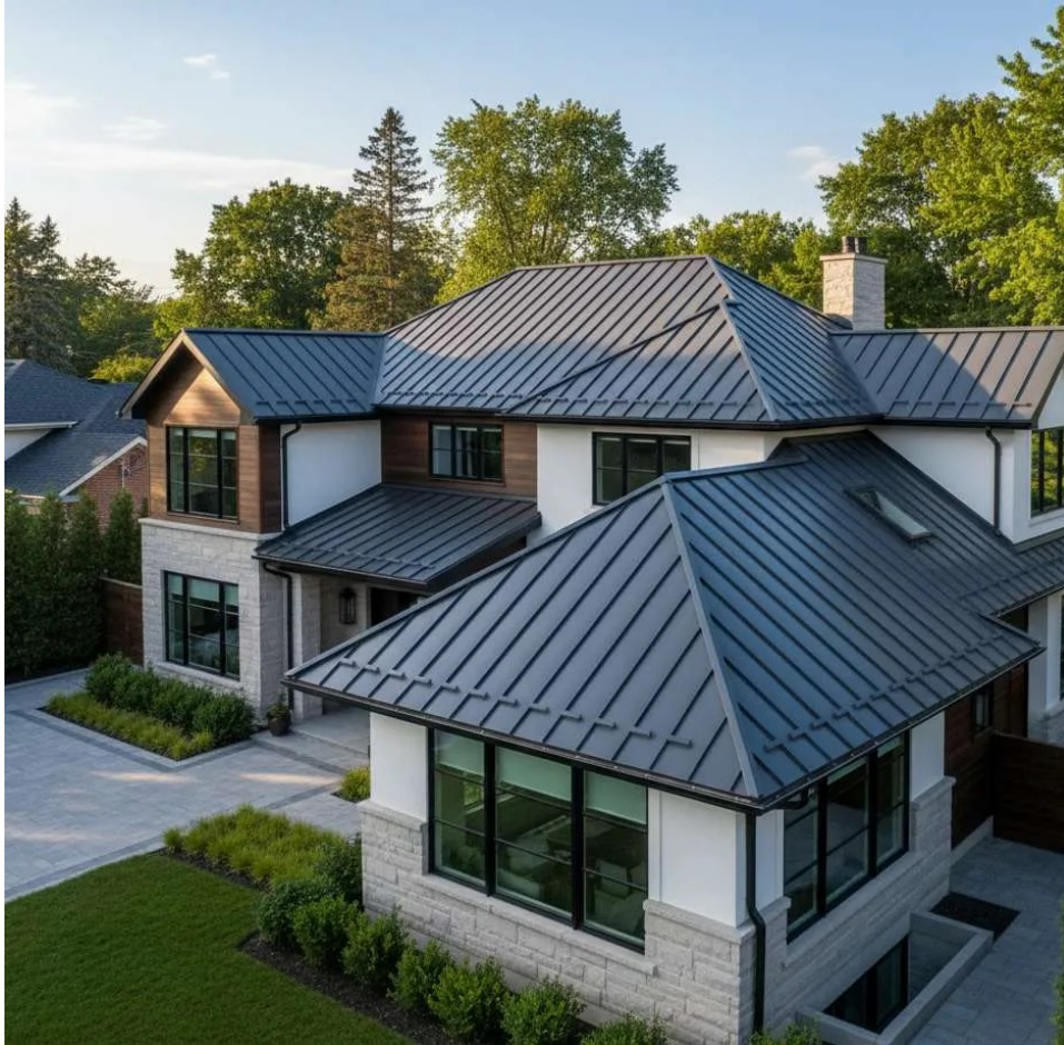
Standing seam metal roof on a Southern California home.
