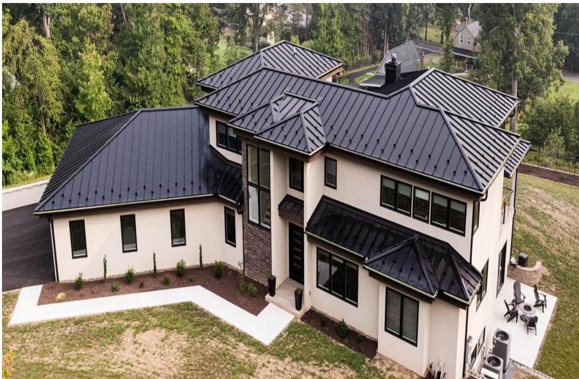
Standing seam install on a Hidden Hills estate, designed for wildfire exposure, wind, and architectural impact.
