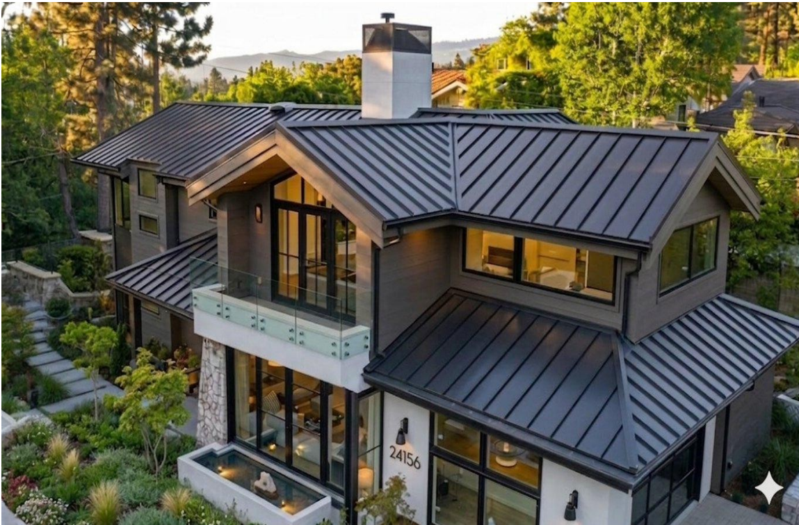
Standing seam on a Beverly Hills modern, the roof has to be invisible and perfect at the same time.
