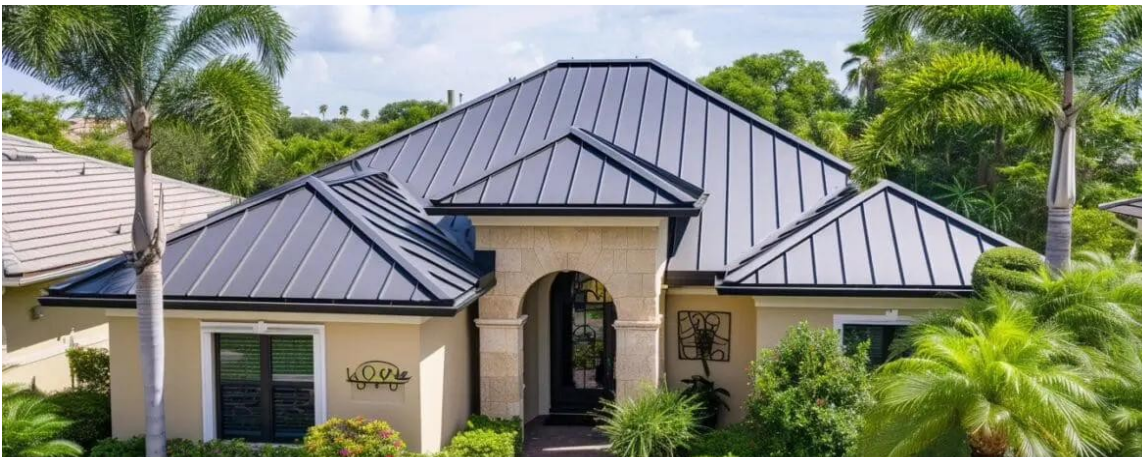
Exposed-fastener "5V" roofing, note the visible screws every few inches. Standing seam hides all of these.
