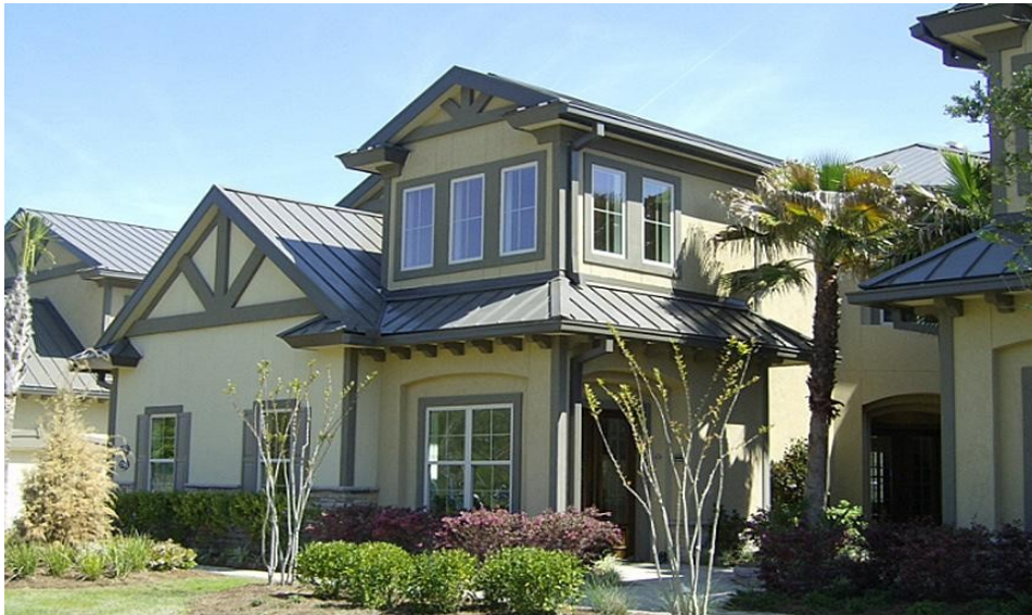
Sheffield Metals, a representative architectural standing seam installation.
